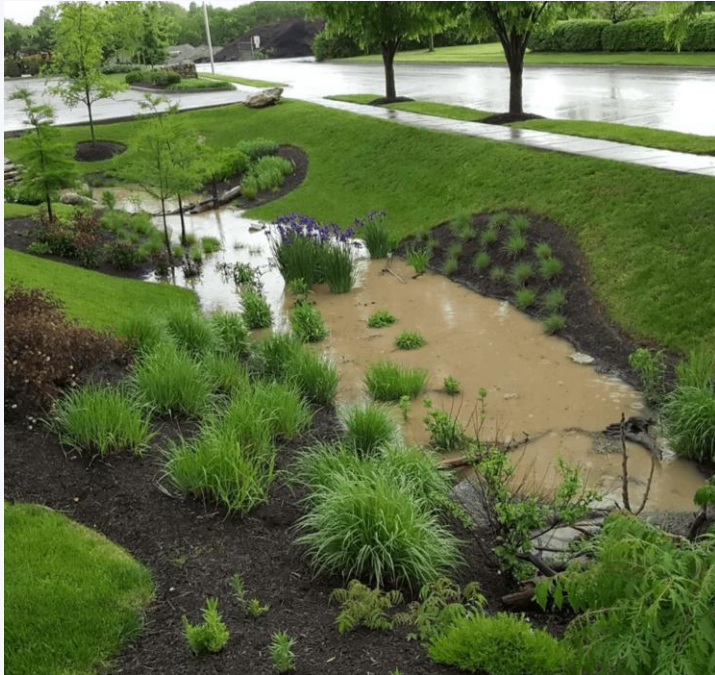
A bioswale integrates into the landscape, managing water while providing aesthetic value.
