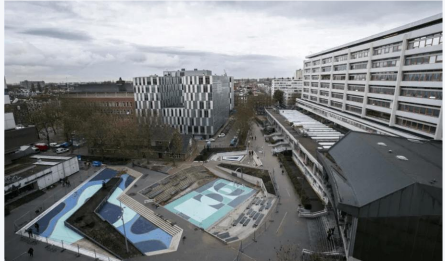
Rotterdam Water Square: A playground that transforms into a retention basin during heavy rain.
