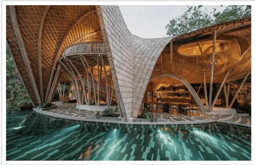
The "Heart of School" building: A masterpiece of bamboo engineering that works with tropical climate forces.
